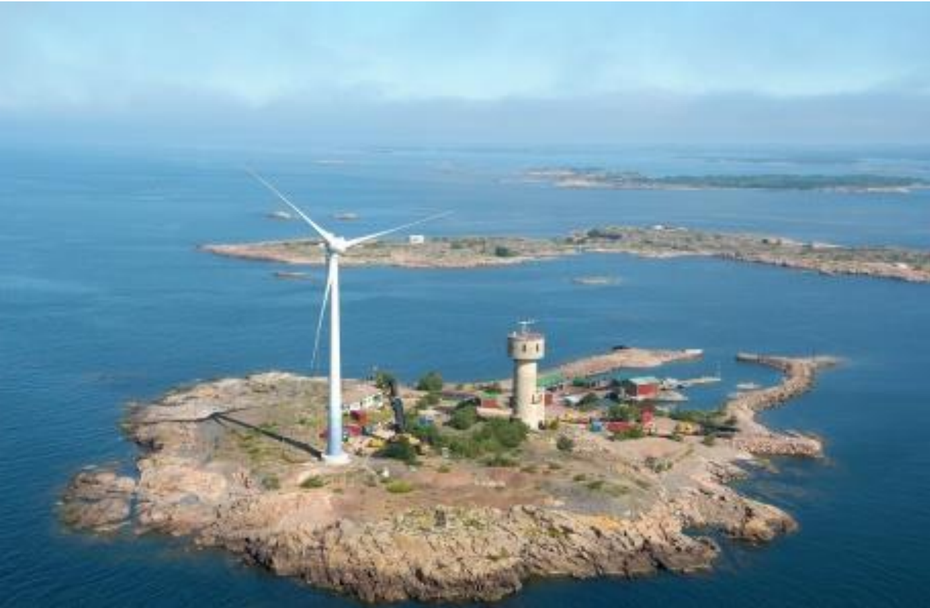
Windpower station on the island of Lilla Båtskär in the Åland archipelago. Photo: Kraftnät Åland Ab; Source: Nordic Investment Bank
